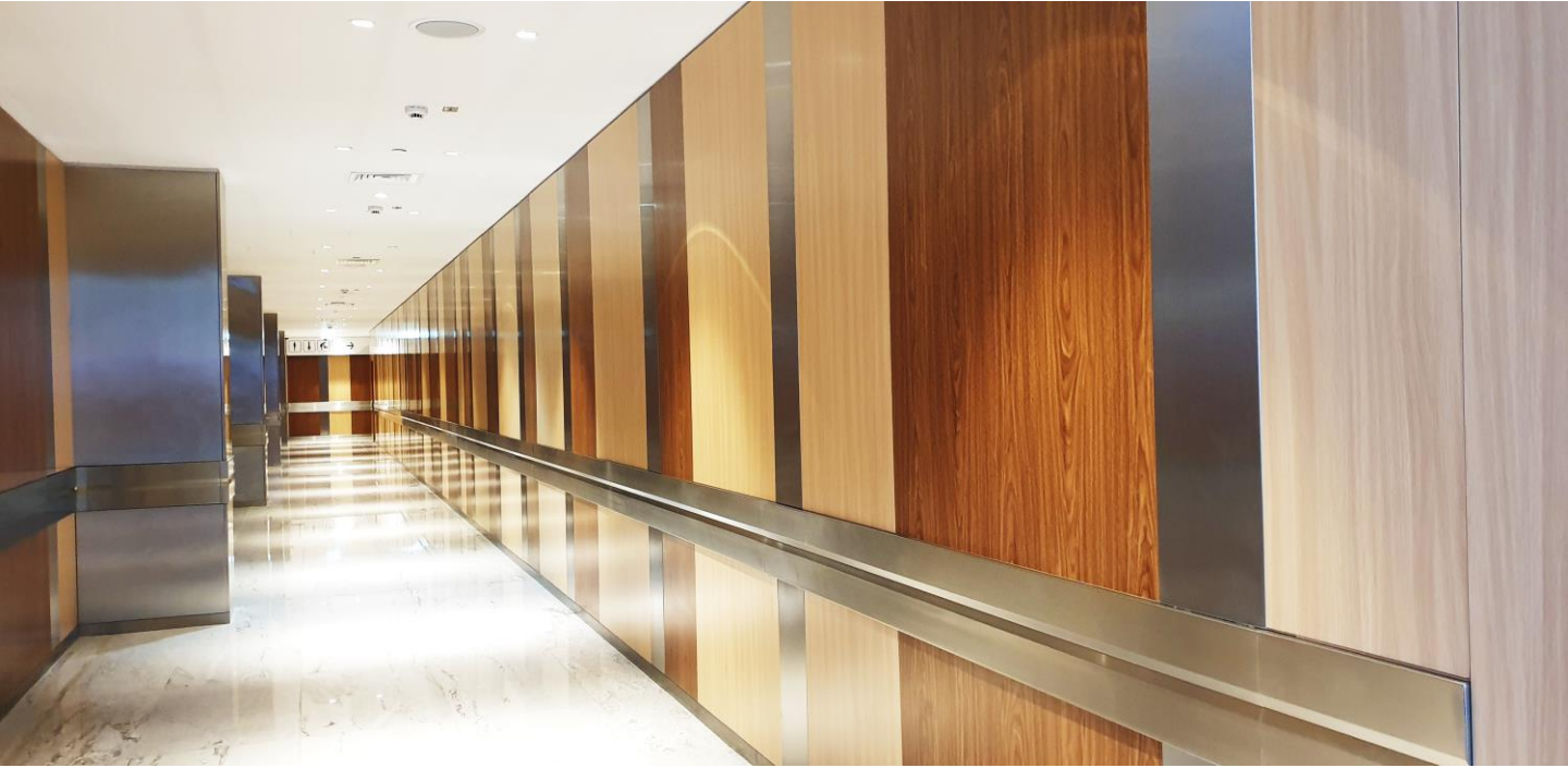
Right side: SS crash rail wall.
