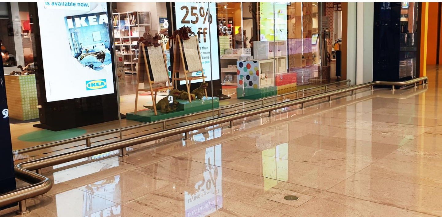
SS Guard rail along the glass wall for protection.
